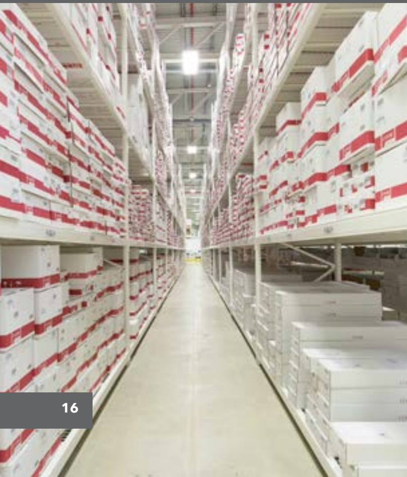
Cook Distribution Center
